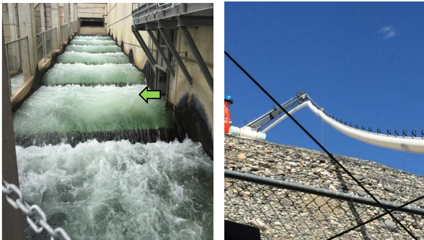
Figure 5. Left panel is the last 15.5 vertical feet of the Priest Rapids fish ladder. The green arrow indicates the location through which control fish pass from the calm water channel to enter the fish ladder. Right panel is a portion of the 180 ft long WFTS tube with the 40 ft climb used in the head to head sub-study. The WFTS was temporarily installed, used and removed all within 8 hrs. on a single study day.
